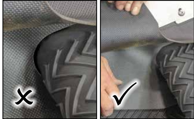
Fig 30 - Corner flashing must fit tight around the belt
